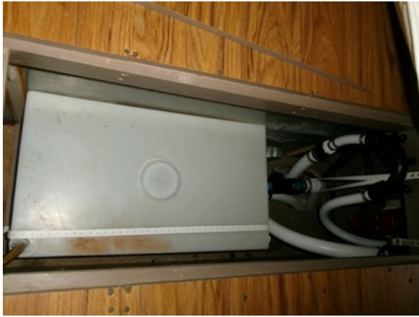
What lurks under the aft cabin master berth.
