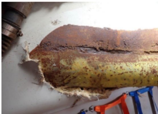
Figure 2: Severely corroded remnants of compressed air cylinder shell. Note the distinct line of deep pitting.
